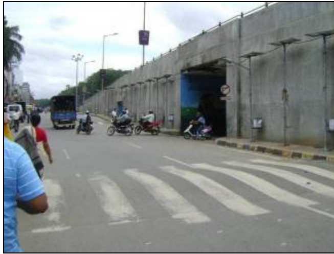
Plate 4-13 View of at-grade service road
