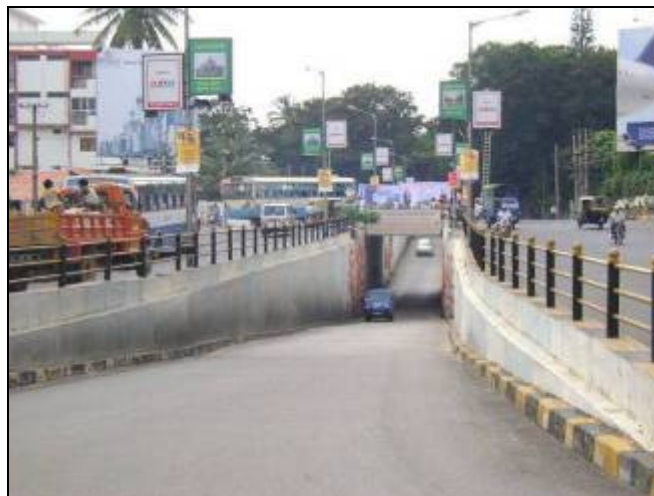
Plate 4-10 View of Underpass at Cauvery Theatre Junction
