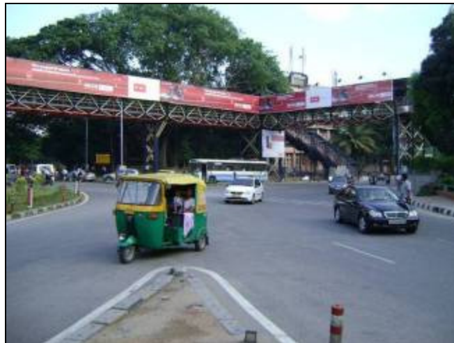
Plate 4-3 Pedestrian Skywalk at High Grounds Junction
