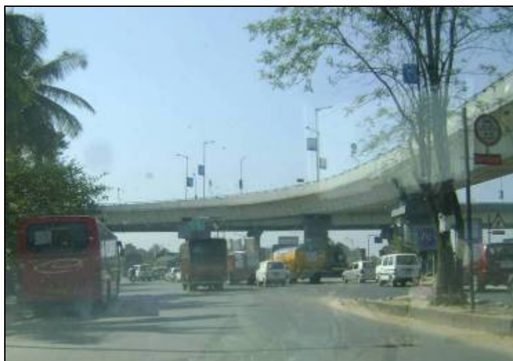
Plate 4-18 View of at-grade road at Hebbal Junction
