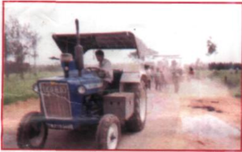
Surface cleaning using air compressor
