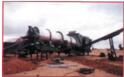
Erection of Hot Mix Point
