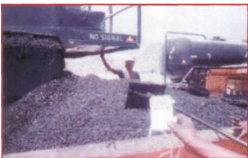
Temperature check for the mix
