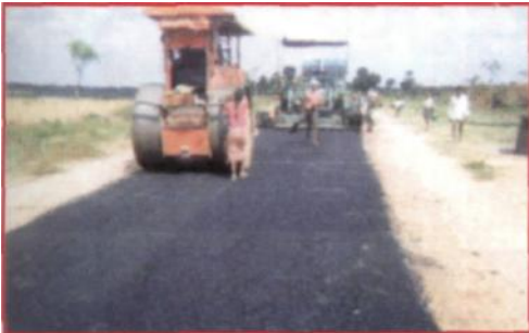
SDBC in progress
