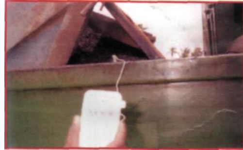
Temperature checks for the mix
